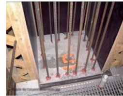
Extension of columns via splices
