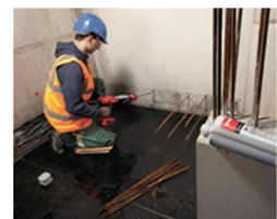
Slab to wall via splices or end anchorage
