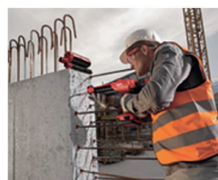
Wall extension via splices
